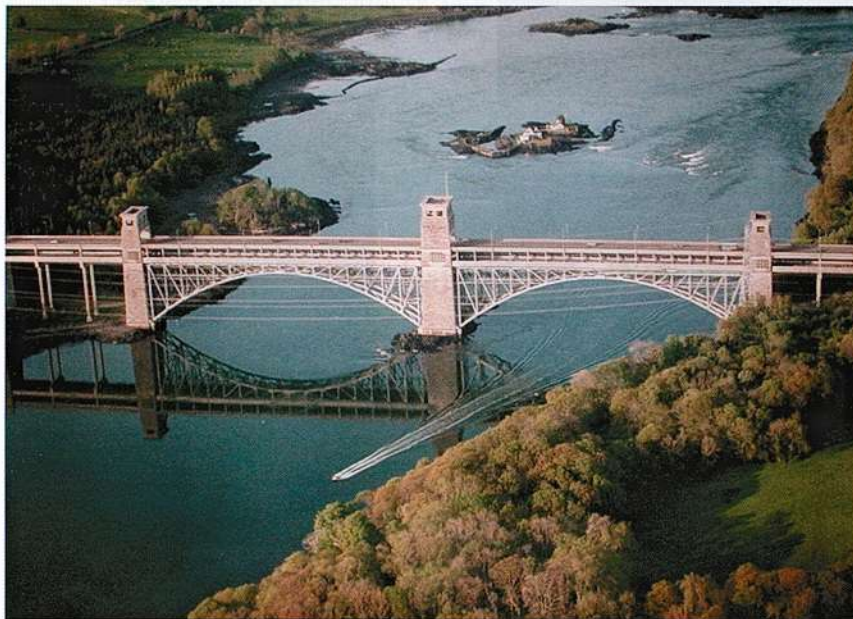
Britannia Bridge-Menai Straights
